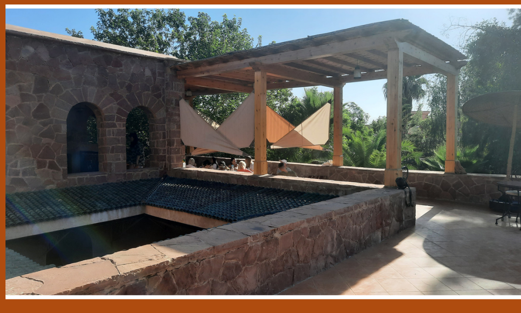
Roof top terrace dining
